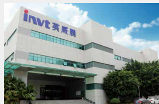
Shenzhen Fuyong Industrial Park
